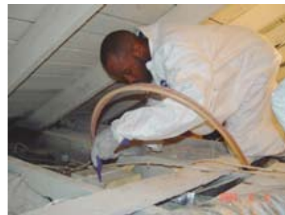
Two-part foam insulation. Credit: Alex Moore, www.waptac.com
